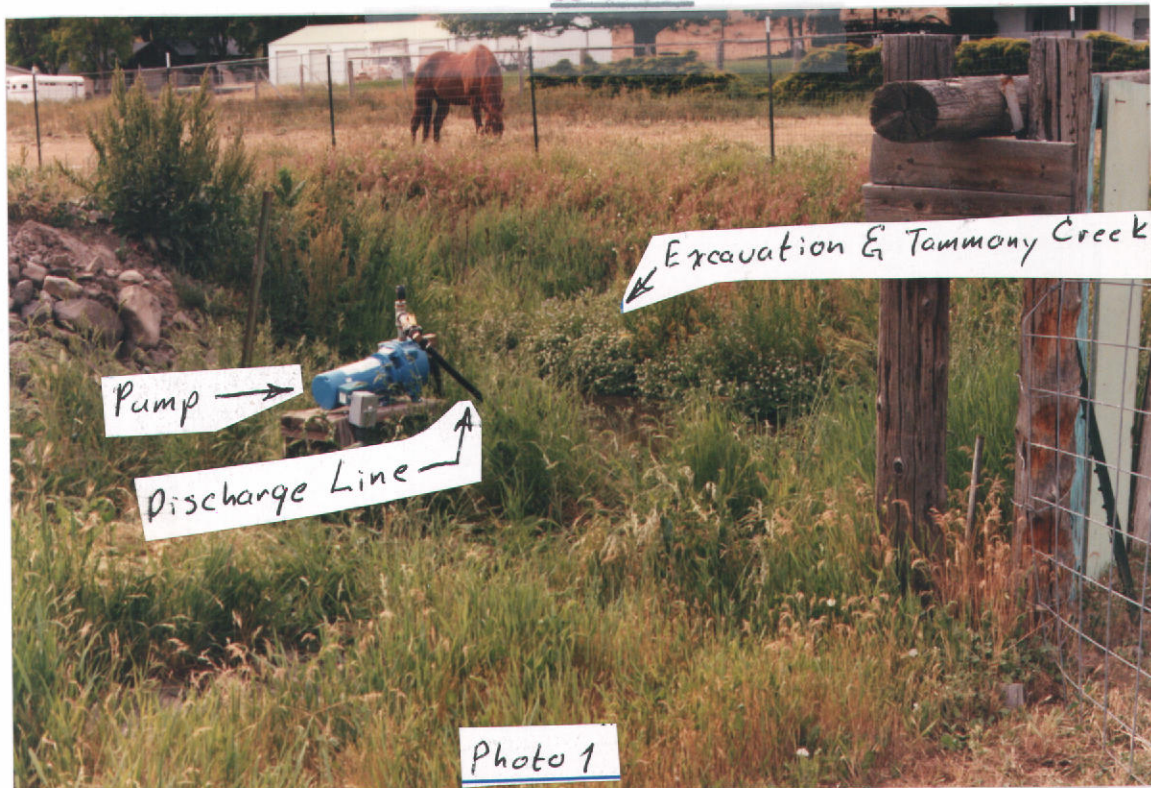
Photo 1. Showing pump placement in Tammany Creek.
