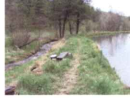
LEVEE BETWEEN LARGE POND AND STREAM
