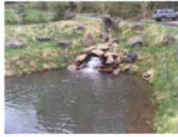
INLET TO LARGE POND
