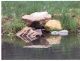
OUTLET FROM LARGE POND
