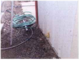
disconnected pipe for filling pond
