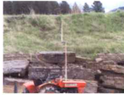
pipe for filling pond
