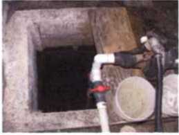
Storage box inside Outbuilding
