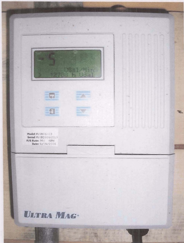
Figure 6: Digital Readout for McCrometer UltraMag flow meter
