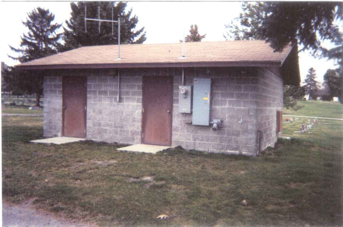
Figure 6. Photographs of the Caldwell Well #4-B pump control house. The upper view shows the Well #4-B in the background and looks east to the north and west walls of the control house. The two well flushing lines are visible exiting the pump house into a grated drain. The lower view is of the south side of the pump control house showing access.
