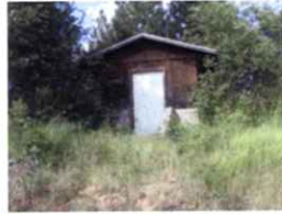
WELL HOUSE IN USE
