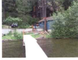
POINT OF DIVERSION
