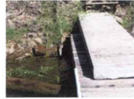
POINT OF DIVERSION
