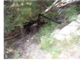
92-10023 Reservoir overflow to unnamed stream.JPG
