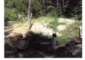
92-10023 Reservoir & POD at rear post.JPG
