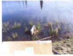
POINT OF DIVERSION INLET
