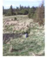
POINT OF DIVERSION OUTLET
