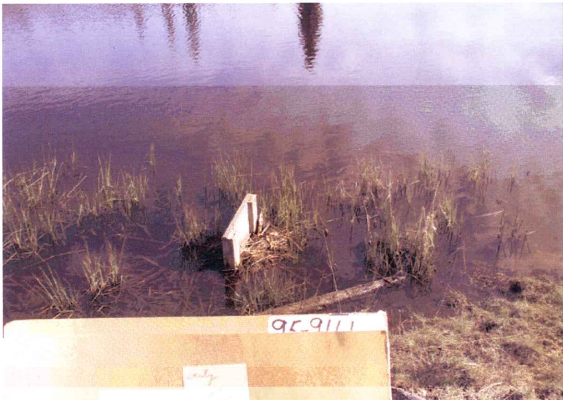
POINT OF DIVERSION INLET
