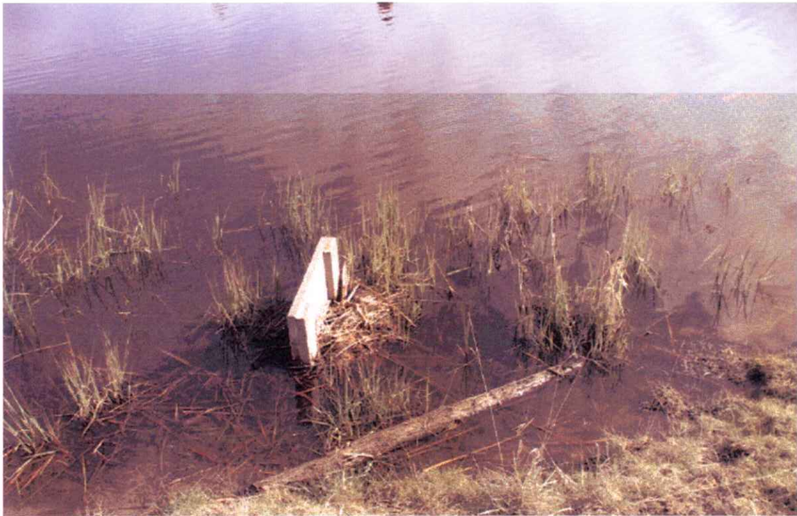
POINT OF DIVERSION INLET
