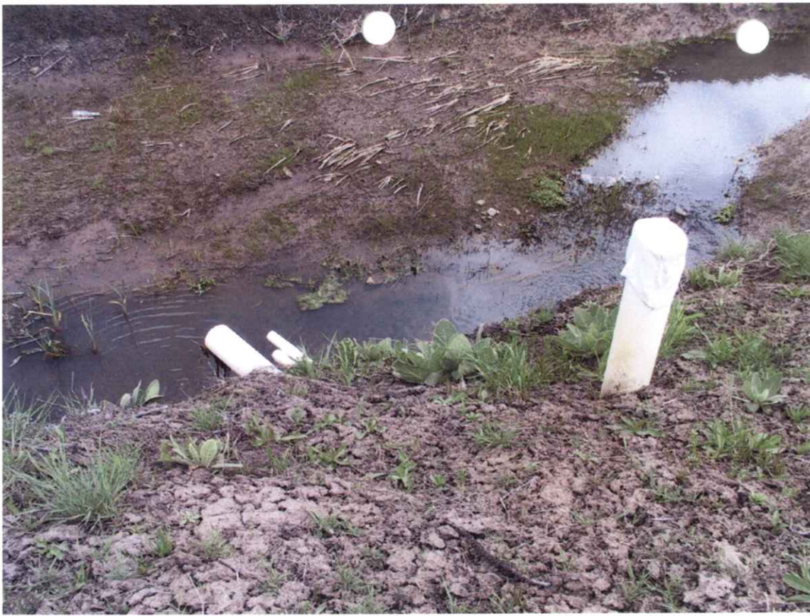
outlet to stream
