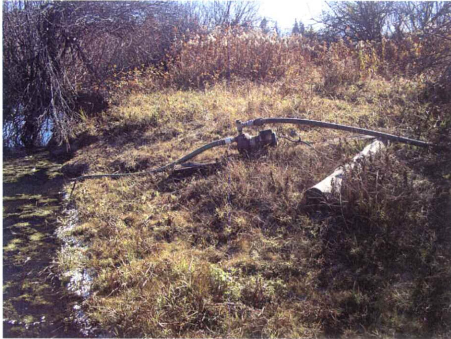
P/D: 2 hp pump on unnamed stream Picture of 8 hp gas pump used for river diversion in file 65-22904
