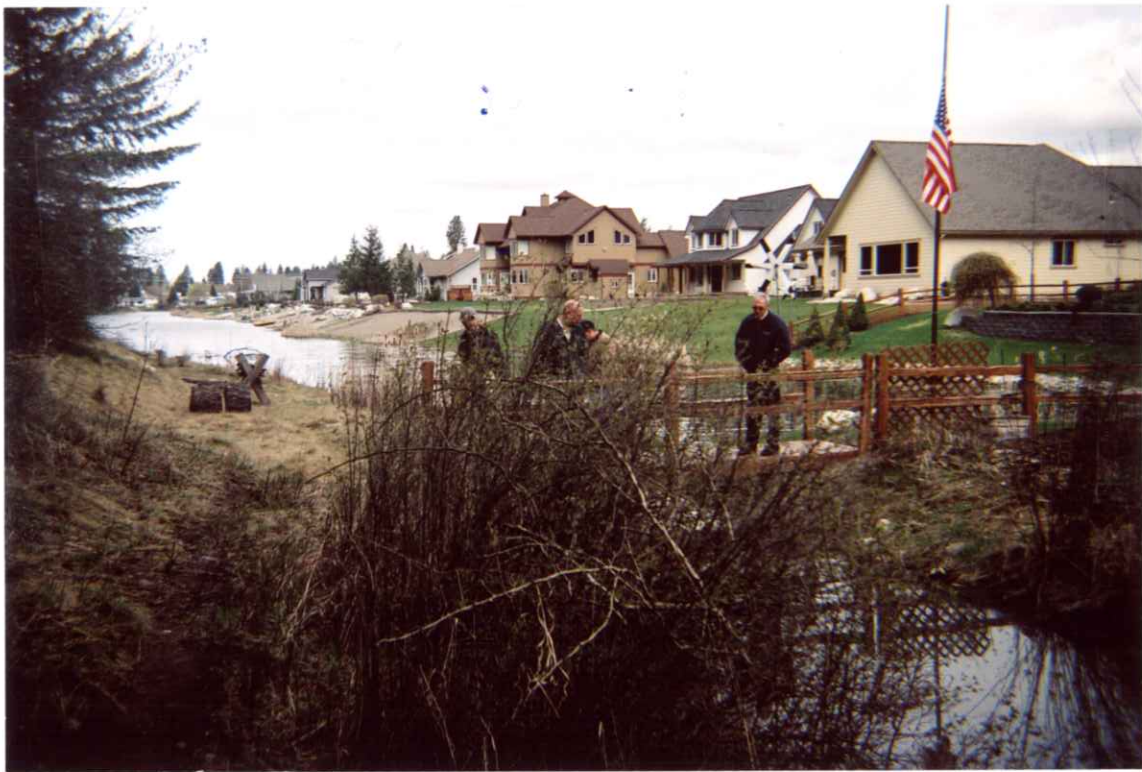
Inlet to Pond
