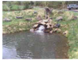
INLET TO LARGE POND
