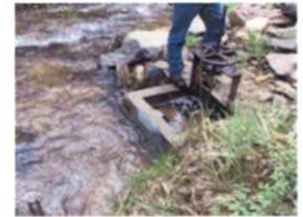
POINT OF DIVERSION
