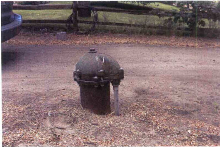
East facing view of well
