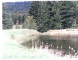
small pond and dam
