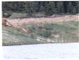
outlet for large pond
