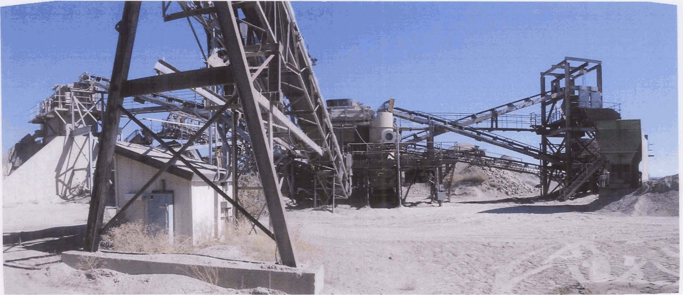
Additional facilities. Truck fill station at right.
