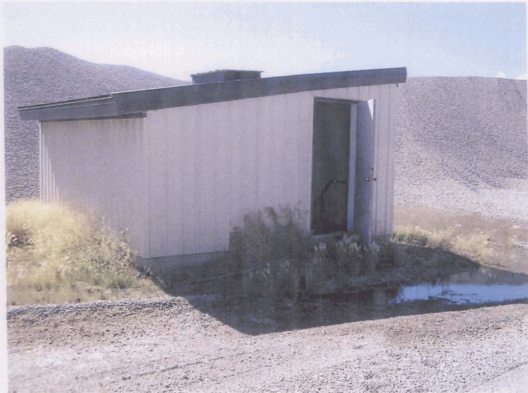
Shop Well shelter
