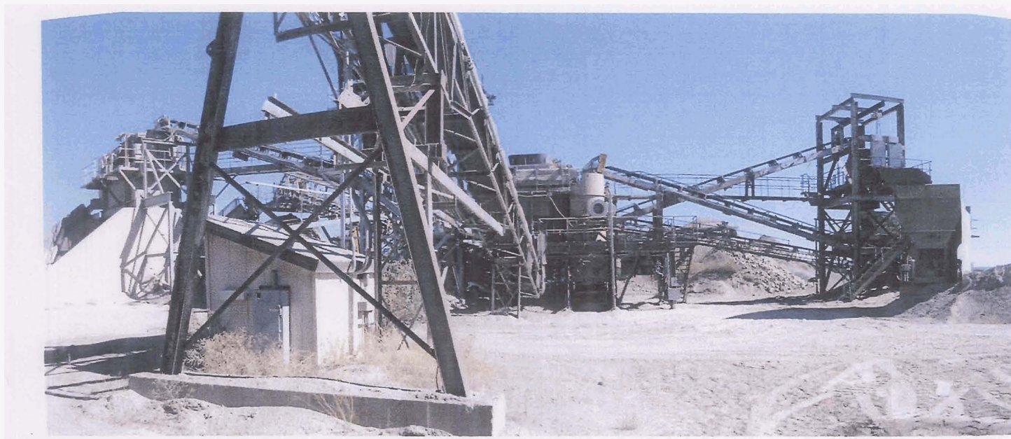
Additional facilities. Truck fill station at right.
