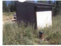
WELL AND PUMP HOUSE
