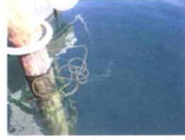
POINT OF DIVERSION
