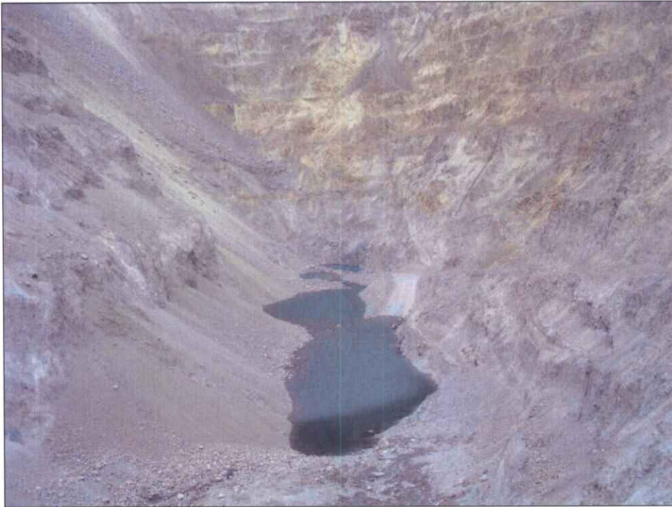
Photo 1: Low-elevation mine pit sump. The 140-hp Flygt submersible pump is located at the far end of this pond. The pump was not accessible during field exam due to excessive falling rock.
