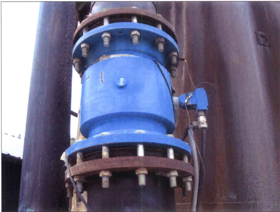
Photo 5: Krone 10-inch Altometer Magnetic Flowmeter.
