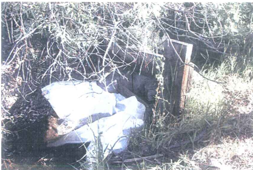
Headgate at POD 74-54 6/28/07
