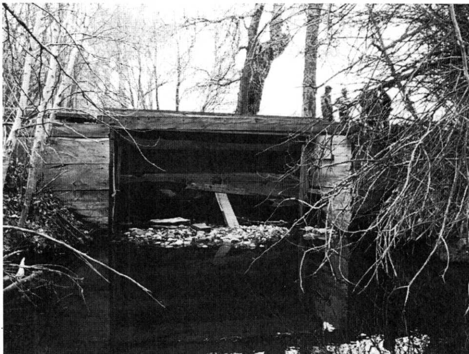
Figure 3: Big Timber 2 Diversion from below.
