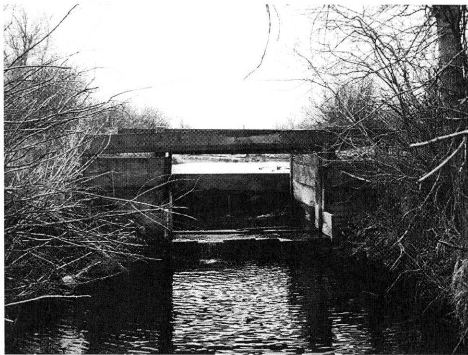
Figure 5: Intercept structure looking upstream the Big Timber channel 5/16/05.
