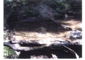
POINT OF DIVERSION
