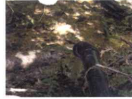
PLANT RUNNING AT 23 GPM
