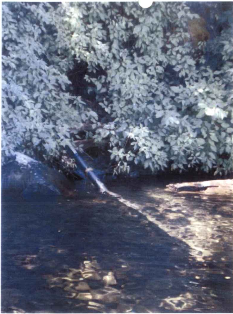
95-8817 water line into lake
