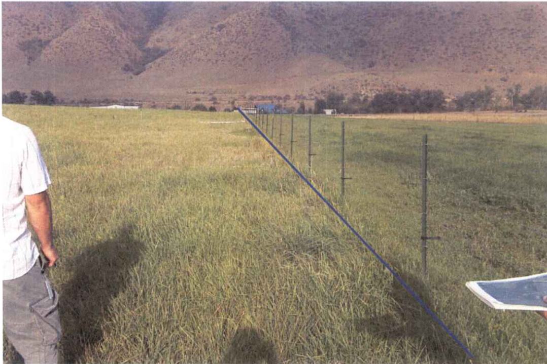
- POU, looking from NE corner down northern boundary. Blue line represents underground supply line.
