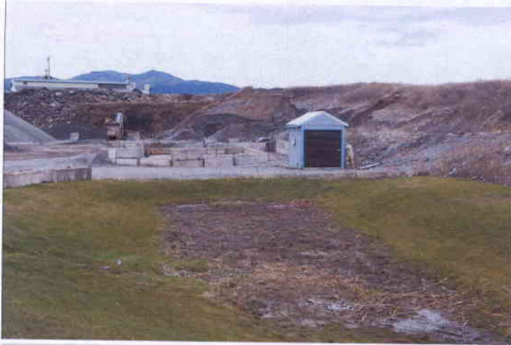
Production well building
