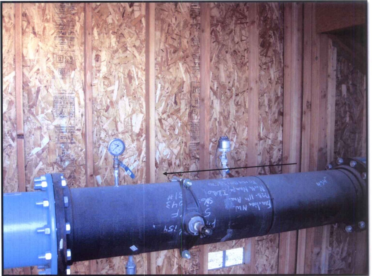
Photo 3 - Delivery from well head
