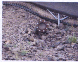
SYSTEM CLEAN OUT
