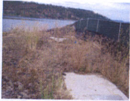
POINT OF DIVERSION
