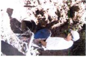
92-10008 POD in trench
