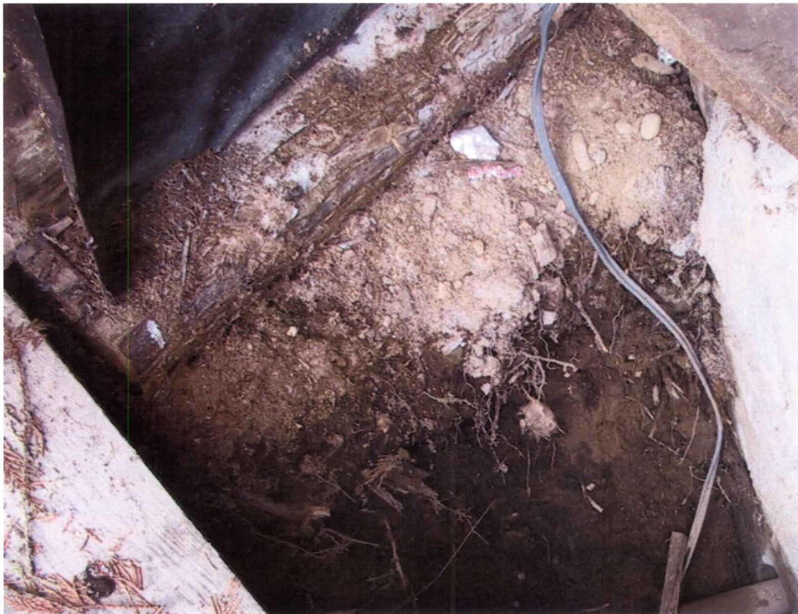
Pipe Running To House
