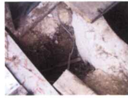
PIPE RUNNING TO HOUSE
