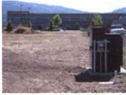
IRRIGATION HOOK UPS EVERY 50 FT ALONG PR...
