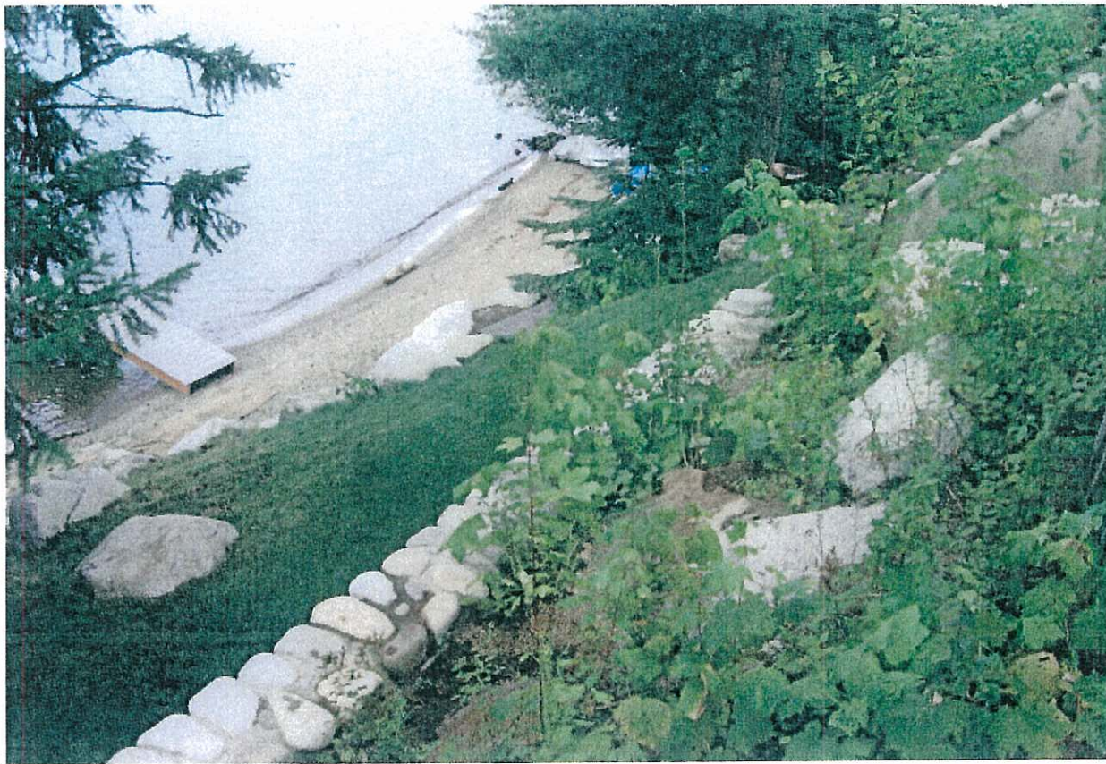
95-9259 Front Irrigation & Drain ↑
