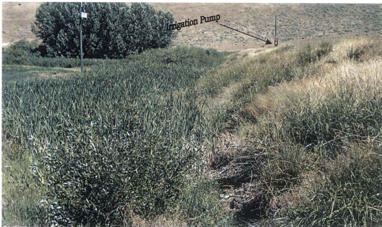
Photo #3:Downstream slope and toe of the main embankment, from the south.
