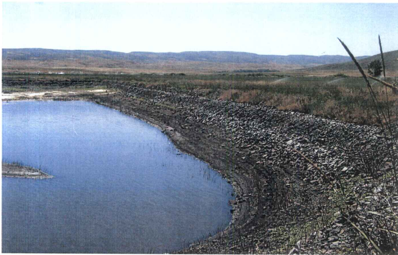
Photo #1: South dike upstream slope- good.
