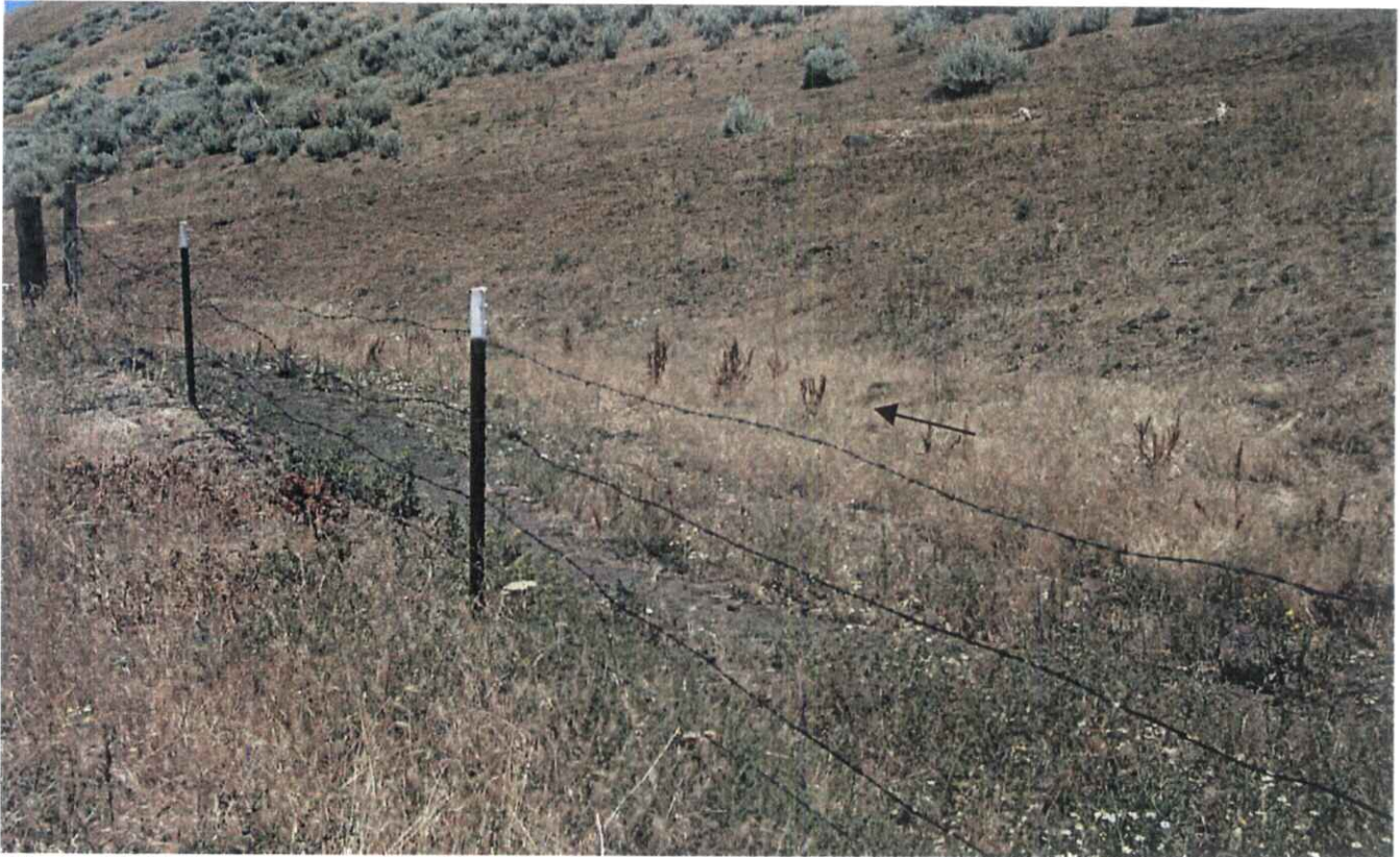
Photo #5: Spillway channel looking downstream.
