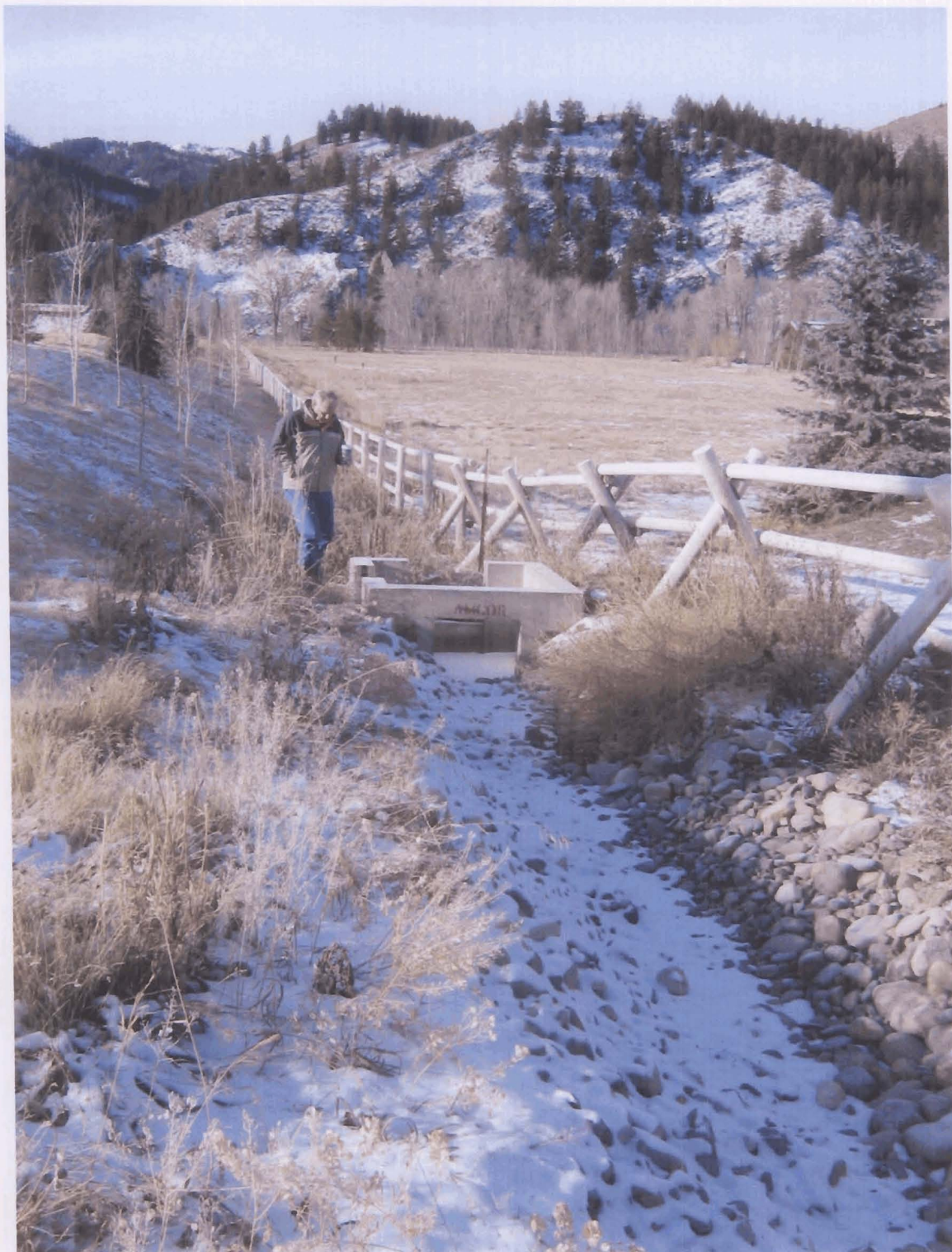
FIGURE 2 Diversion structure and weir from Eagle Creek Irrigation Co. ditch.
