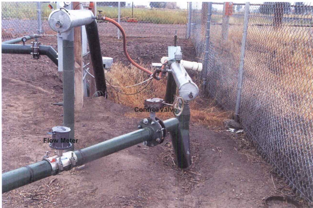
Diversion works: Flow meter on line from well, ground water flow control valve, and Y-pipe joining ground water with surface water from canal in background.
