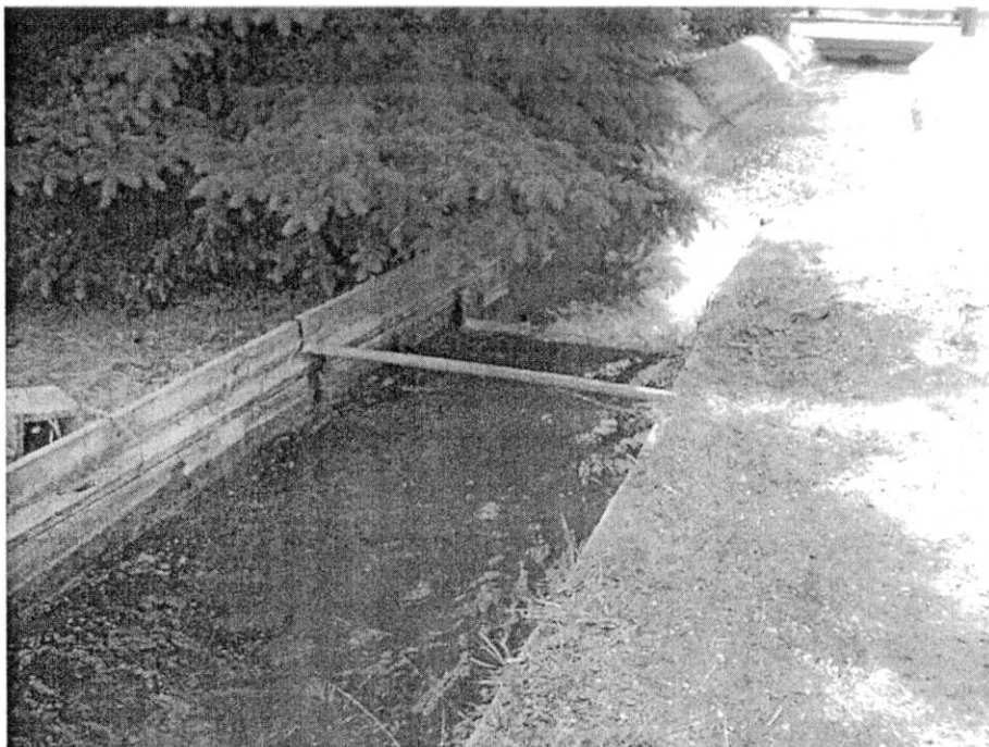
Figure 5 Weir installed downstream from the headgate on Riverton Road
