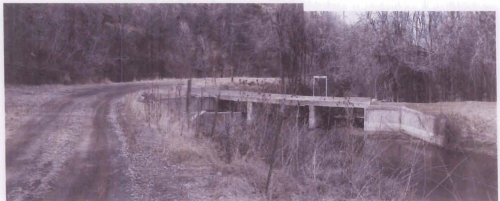
Diversion from Mud Creek below upper power plant diverting water to lower power plant. View looking downstream.
