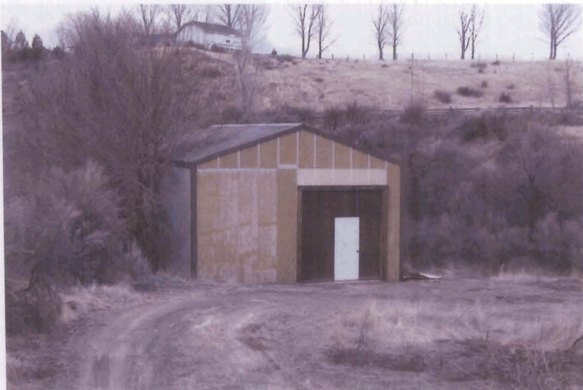
Lower power plant. Generators in building.
