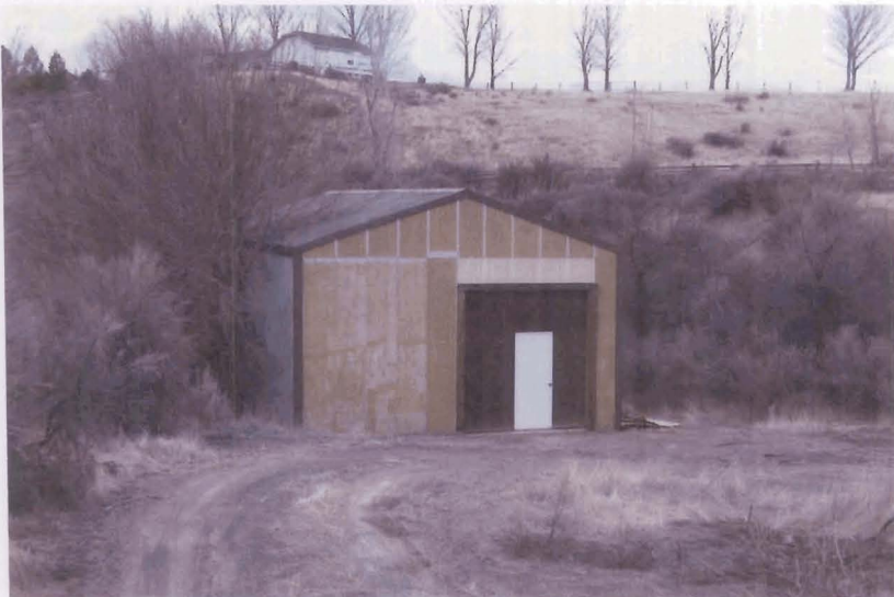
Lower power plant. Generators in building.
