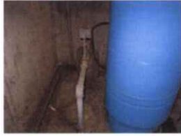
POINT OF DIVERSION
