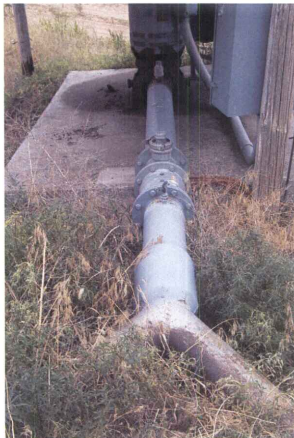
Point of Diversion: View facing east.
