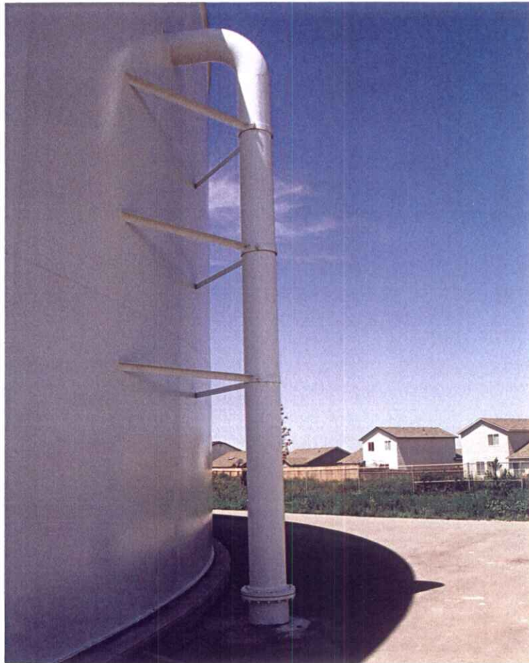
Figure 15. July 11, 2006 photographs of the City of Caldwell's Karcher Reservoir and booster station facility. Lower view looks northwest and shows the 30-foot tall 2 million gallon water storage reservoir with the infill pipe entering the top of the reservoir. The upper photo is a close up of the two pressure gages, inside the pump/control house, indicating the head pressure necessary to pump water into the reservoir.
