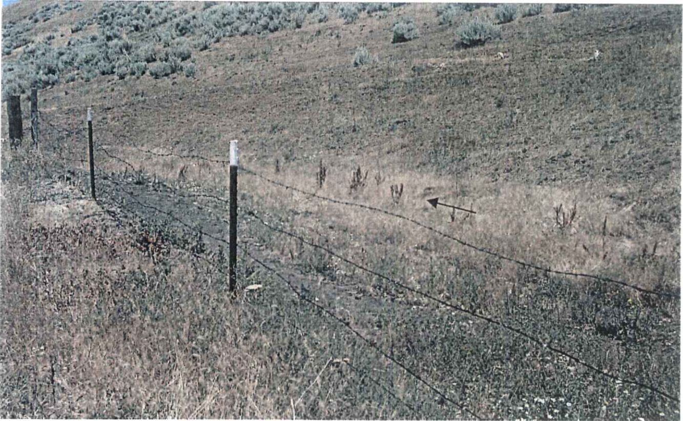
Photo #5: Spillway channel looking downstream.
