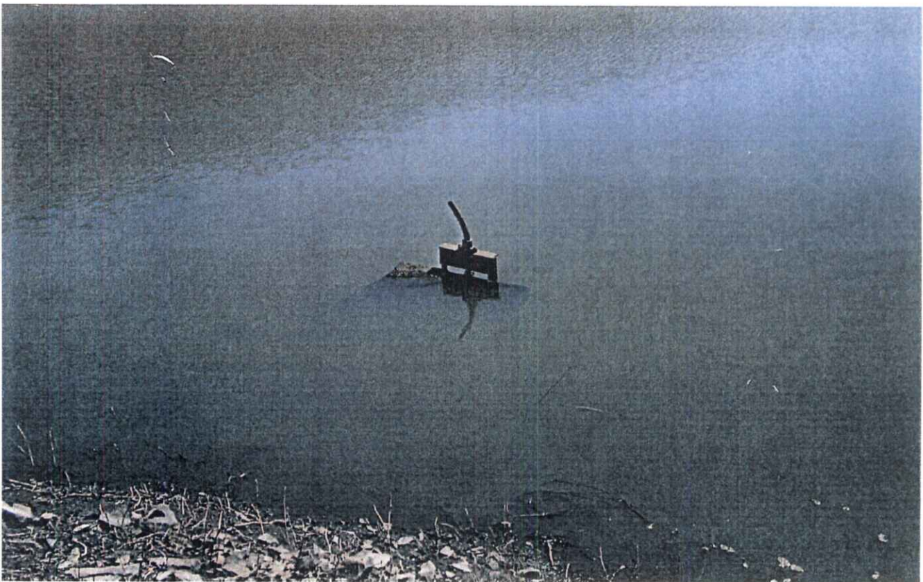
Photo #6: Gate frame sticking up in the reservoir.
