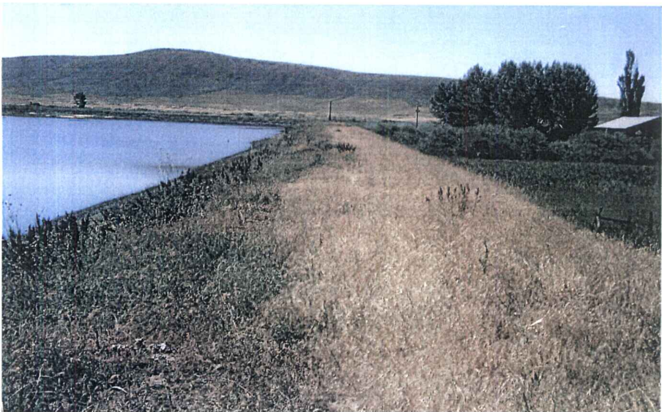
Photo #4: Main embankment crest and upstream slope, good.
