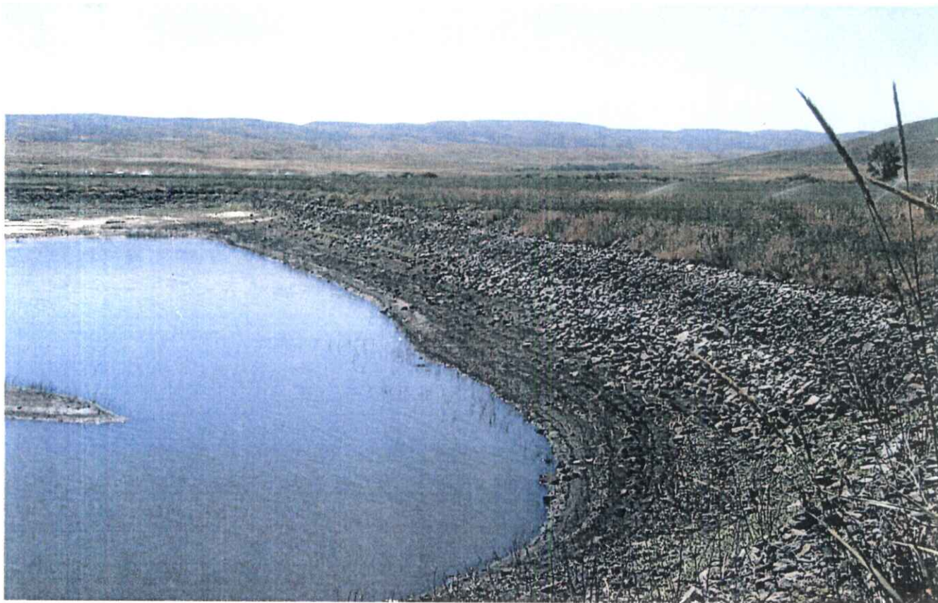
Photo #1: South dike upstream slope- good.
