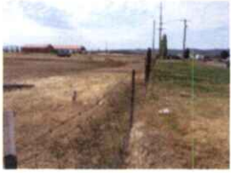
95-8645 Underground line to Prairie AVE.JPG
