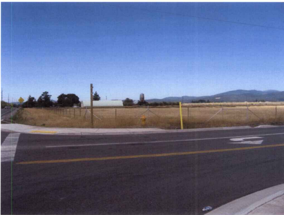
95-8645 Point of Use SE Corner & Hayden Hydrant
