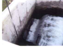
POINT OF DIVERSION
