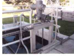
POINT OF DIVERSION
