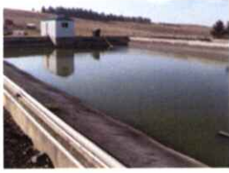
HOLDING POND AND PUMP HOUSE
