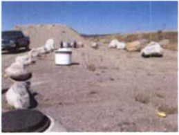
50,000 GAL STORAGE AND 3 BOOSTER PUMPS.JPG
