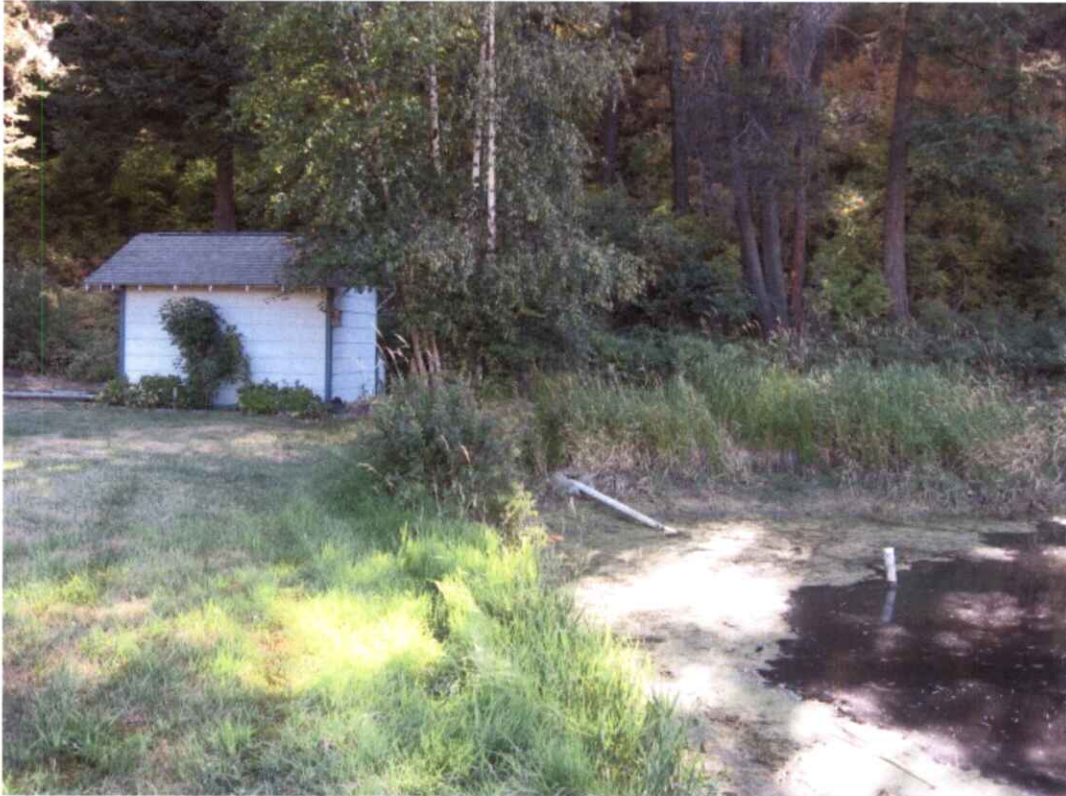
95-9273 Pond Intake Line & Storage BLDG South Side.jpg
