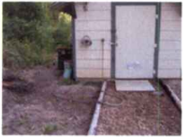
95-9273 Pump Shelter on Left-North.JPG
