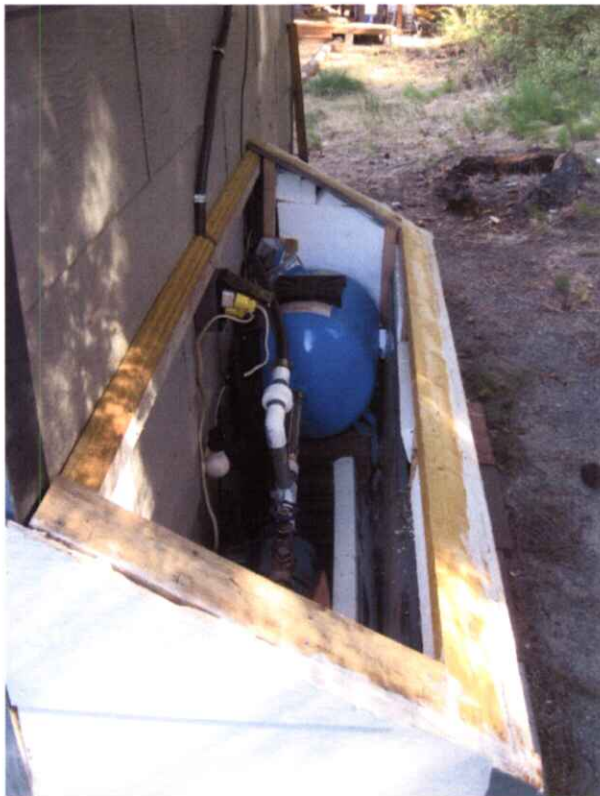
95-9273 Pump House Shelter N Side.jpg
