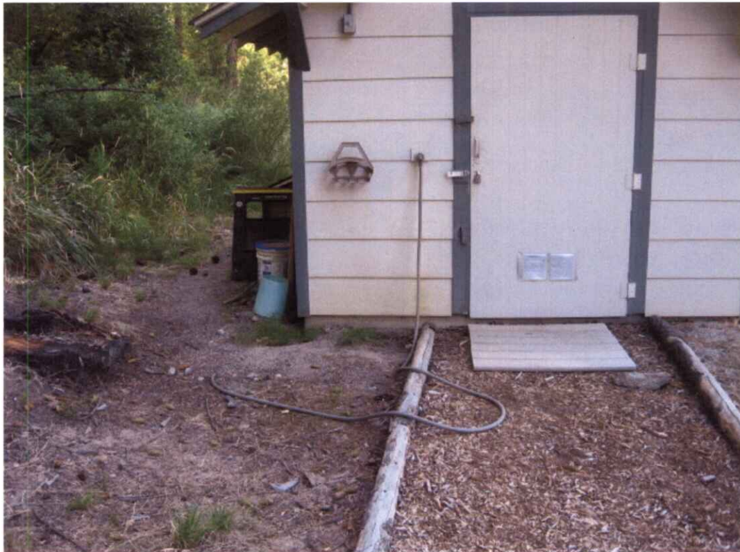
95-9273 Pump Shelter on Left-North.jpg
