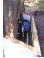
95-9273 Pump House Shleter N Side.JPG
