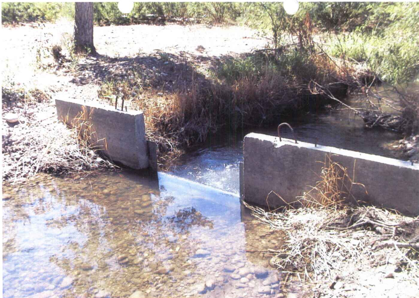
STANDARD CONTRACTED RECTANGULAR WEIR 4' Length Water H: \approx 0.37' = 2.94 CFS
