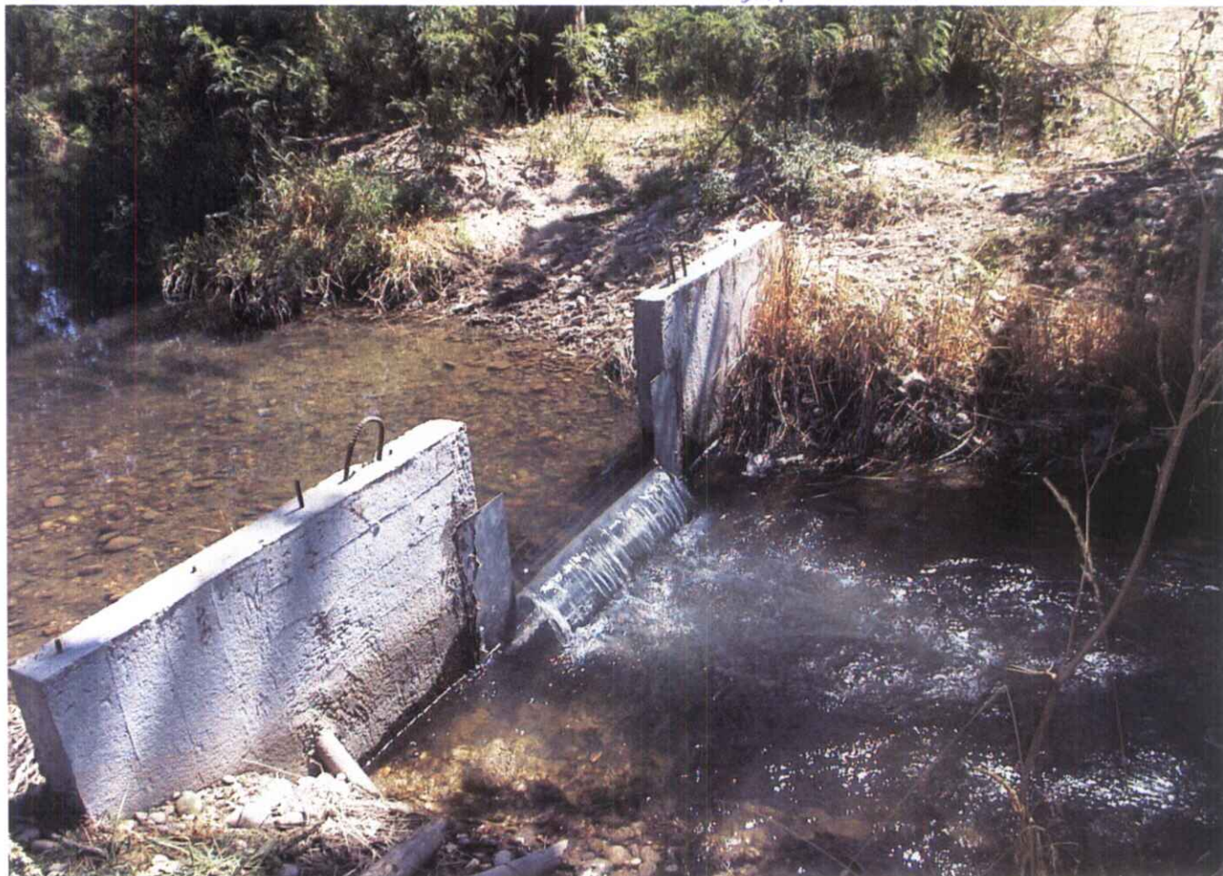
STANDARD CONTRACTED RECTANGULAR WEIR 4' Length Water H: \approx 0.37' = 2.94 CFS
